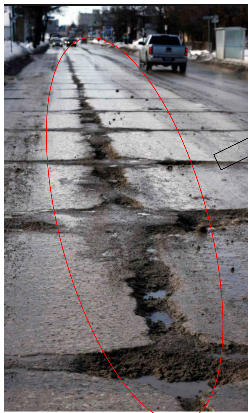
Figure 1. Moisture induced damage to pavement 1
